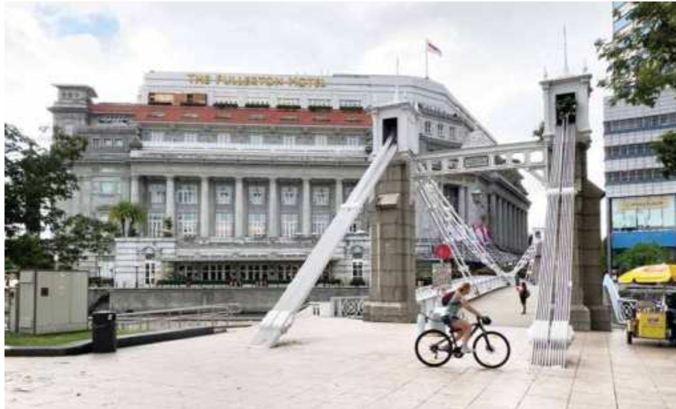
Fullerton Hotel and Cavenagh Bridge, 2023. The old Master Attendant's Office would have been at the river-facing front of today's Fullerton Hotel. Photo by Jimmy Yap.
