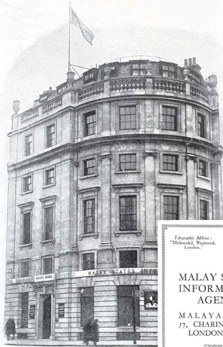
(Above) A sketch of Malaya House in Trafalgar Square, London. The building housed the Malayan Information Agency. Image reproduced from British Malaya: General Description of the Country and Life Therein (London: Malayan Information Agency, 1932), back cover. (From National Library, Singapore, Call no. RCL05 959.5 MAL).
