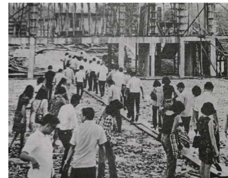
Teachers visiting the Teachers' Centre construction site, 1972. Image reproduced from Mentor vol. 2, no. 6 (October 1972) (Singapore: Singapore Teachers' Union, 1971–), 6. (From National Library, Singapore, call no. RSING 331.881137 M).
