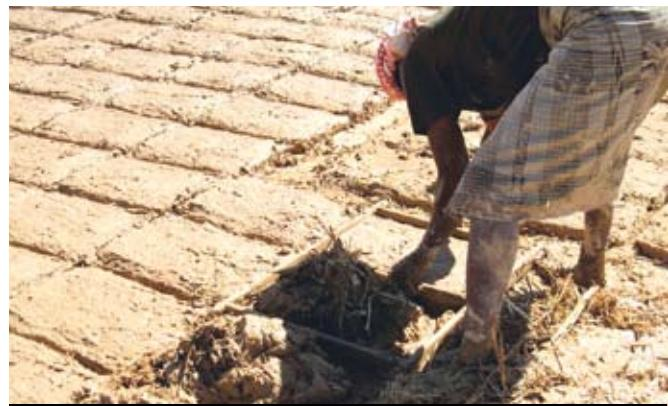
Putting mud mixture into the mould.
