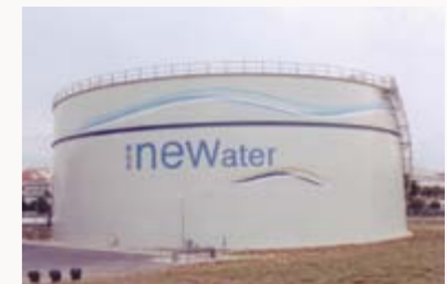
In 2003, the Public Utilities Board developed NEWater, a form of high-grade reclaimed water purified for drinking using advanced water purification technology. NEWater now provides for 30% of the nation's water needs. NEWater facility at Changi, 2003. Source: National Archives of Singapore.
