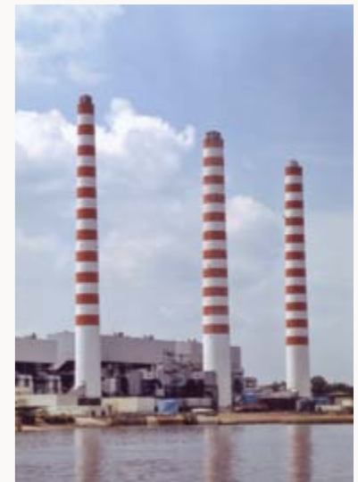
Senoko Power Station is one of several power stations that provides for Singapore's energy needs. Senoko is upgrading its oil-fired steam plants into environmentally friendly gas-fired combined cycle plants that will be among the first in Singapore to use Liquefied Natural Gas (LNG). Senoko Power Station, 1986. Source: National Archives of Singapore.
